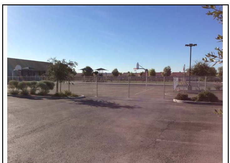
South of Paved Playground
