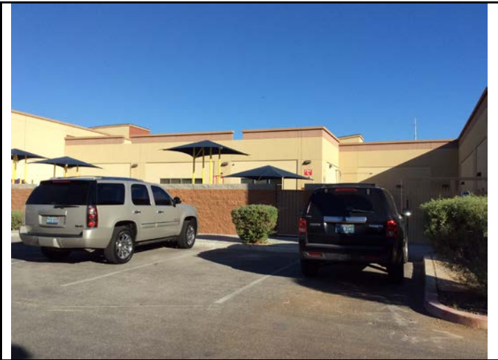
Enclosed Elementary Playground
