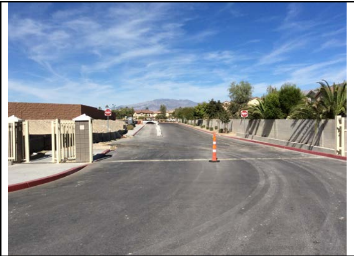
View North - Access Road to Elkhorn Road
