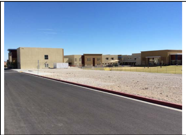
Exterior View – East of High and Middle School
