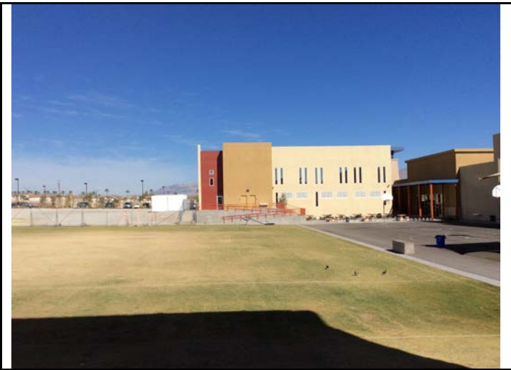
View North - Recreation Field Senior High in Background
